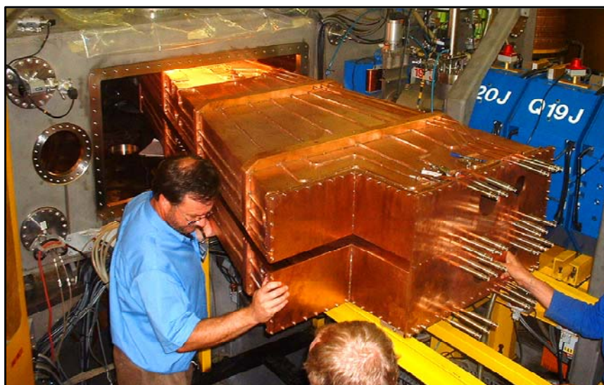
FIG. 4. The flat-top resonator for the SSC during installation through a port in a valley vacuum chamber.
