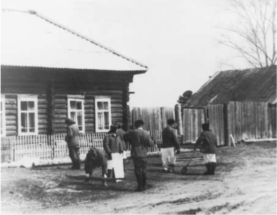
Photo 6. Removal of contamination near a home in Georgievka.
