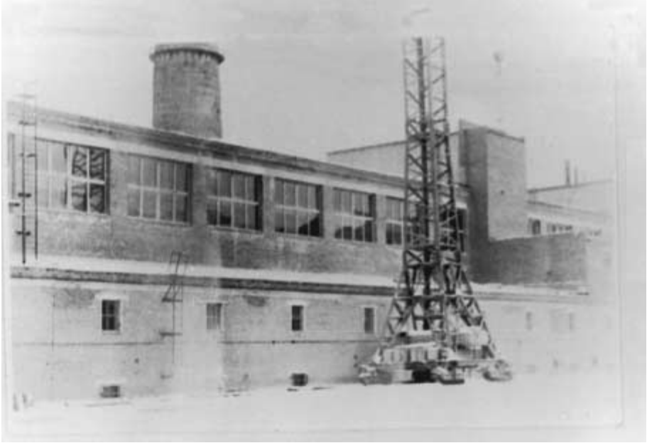
Photo 4. View of Building 201 after restoration.
