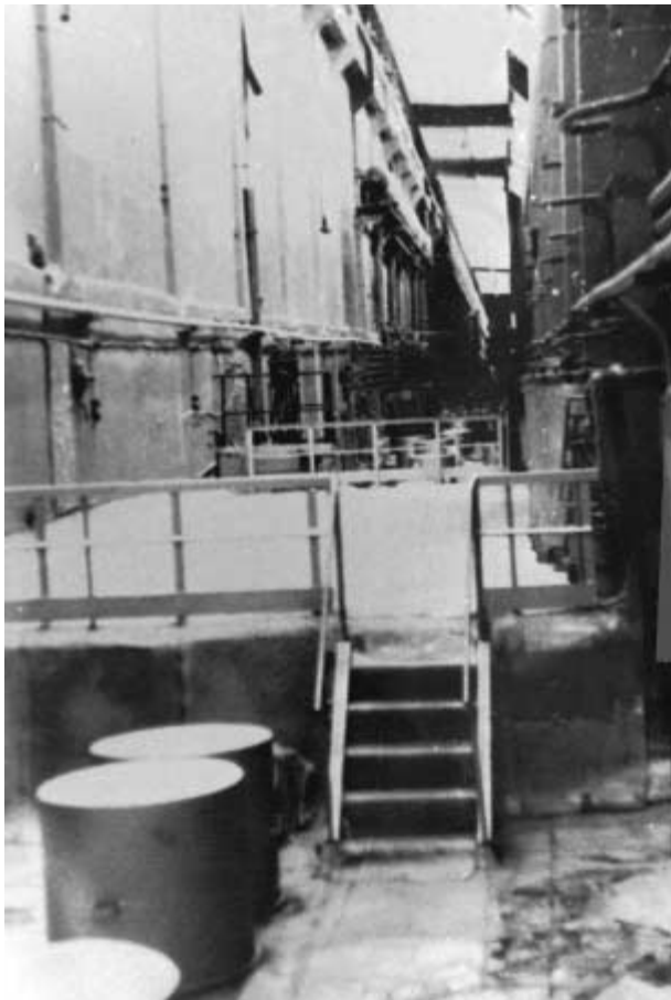
Photo 3. The area around the installation after restoration.
