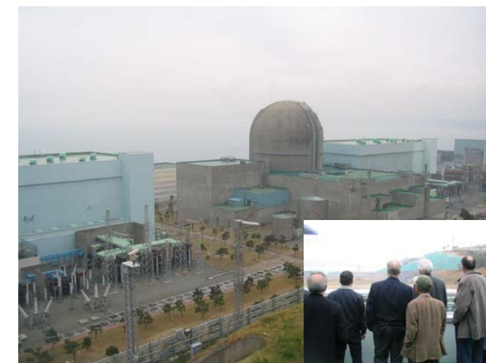
INSAG at the Kori power plant construction site in the Republic of Korea
