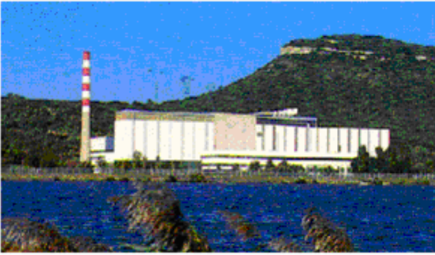
233 MWe Fast Reactor PHENIX, Marcoule, France (courtesy of CEA)
