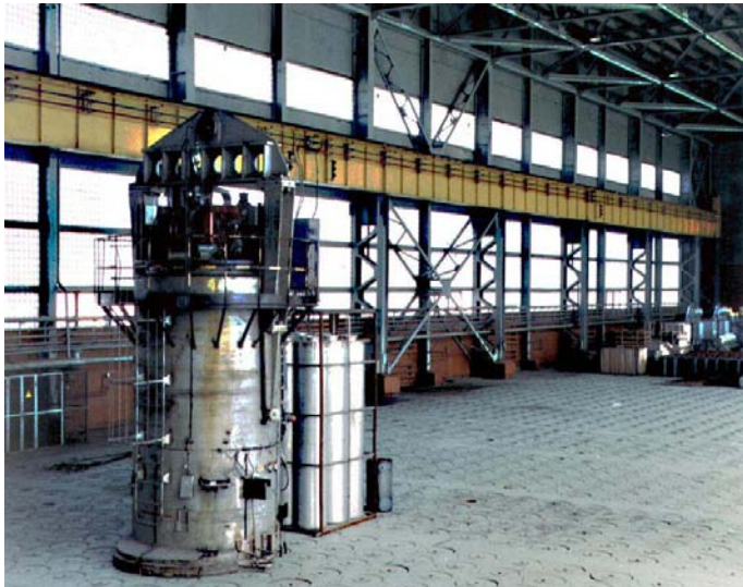
The storage facility for vitrified HLW at PA Mayak with the loading machine at the front. This is where HLW that has been generated during reprocessing of the legacy SNF and heat sources from RTGs are stored.
