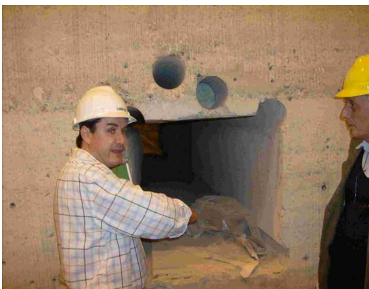
Diamond saw cutting demonstration by ENRESA
