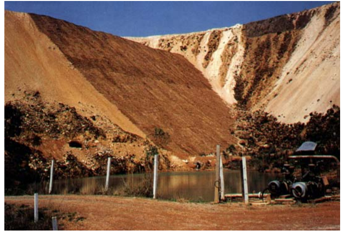
BEFORE: Remediation of an acid-drainage-generating waste-rock dump at the mining site of Pocos de Caldas - Brazil
