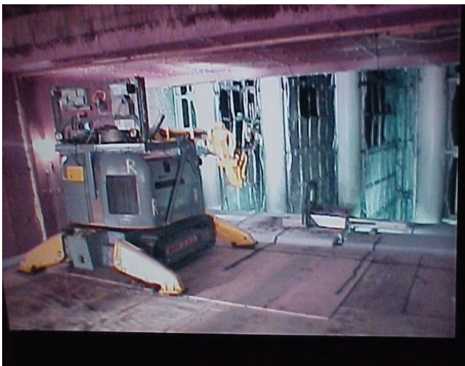
Brookhaven Reactor Decommissioning - 2003
