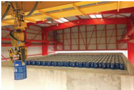
Disposal of Low Level Wastes, Centre de L'Aube, France
