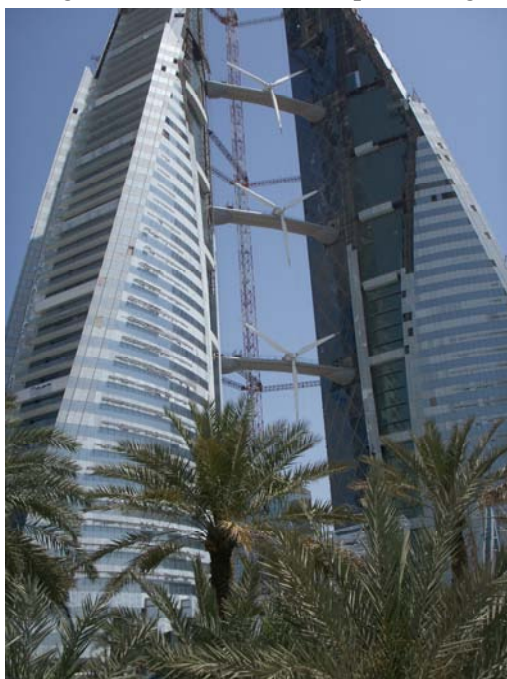
Figure 12: "Wind-tower" with the 3 propellers that provide the electricity for the building.
