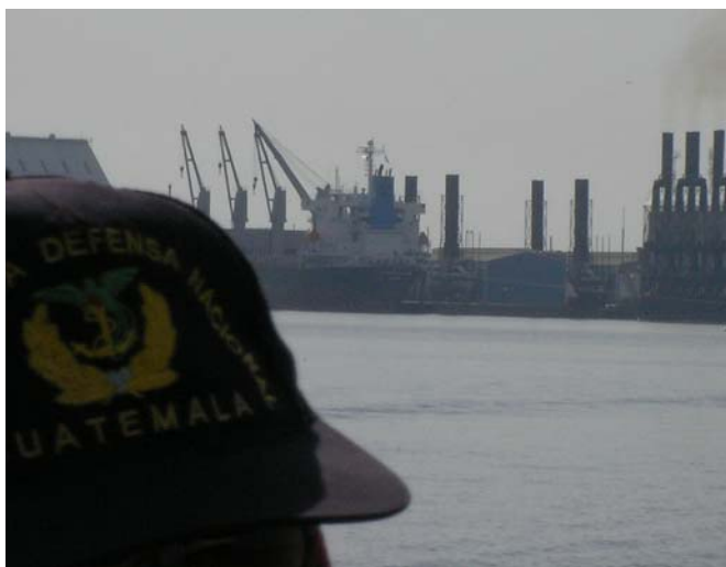
Figure 9: Puerto Quezal (power plant)
