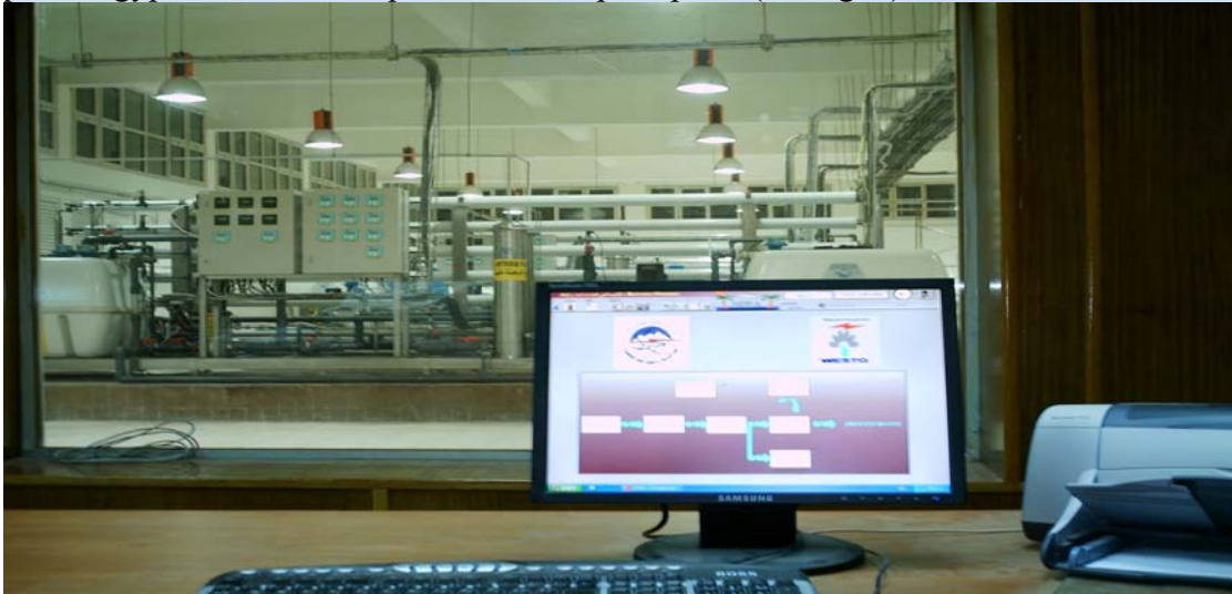
Fig. 1. RO testing Desalination Demonstartion Plant in Egypt
