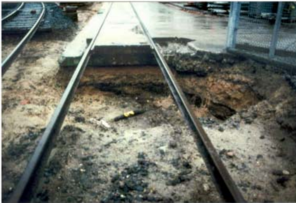
FIG. 13. View after remediation measures at HDR.
