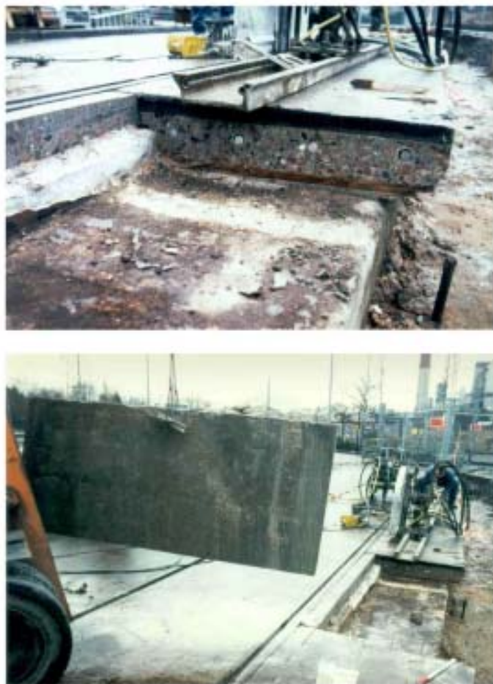
FIG. 12. Segmentation of HDR road to remove contamination.
