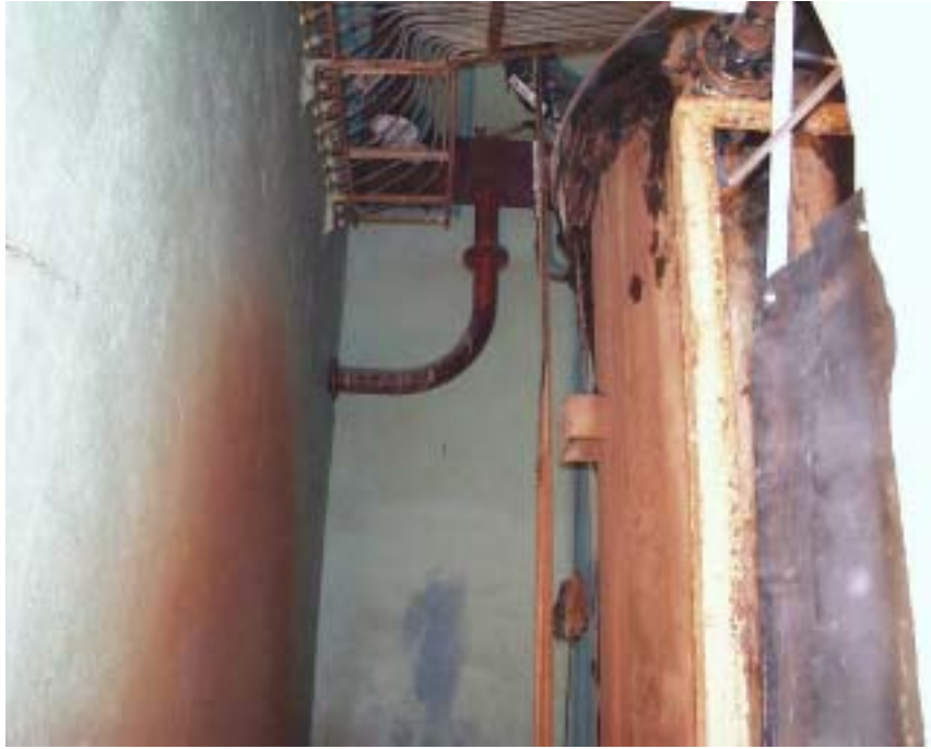
FIG. 16. A-1 NPP, Slovakia, waste treatment system; neutralization tank after decontamination and removal of the insulation.
