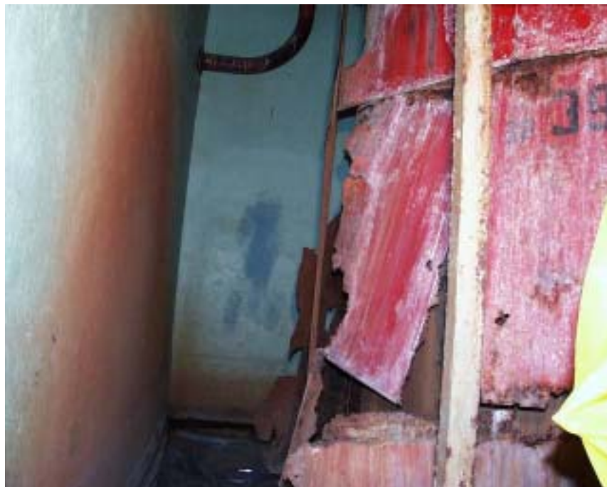
FIG. 15. A-1 NPP, Slovakia, waste treatment system; neutralization tank before decontamination and removal of the insulation.
