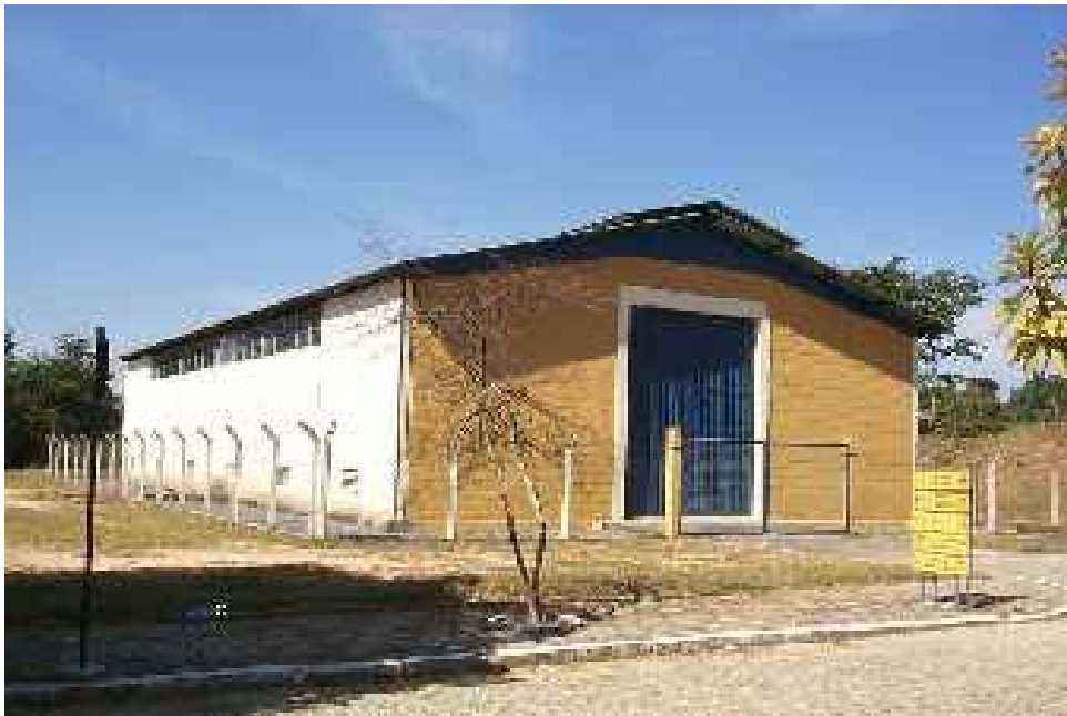
FIG. C-5. Waste storage room at CDTN.
