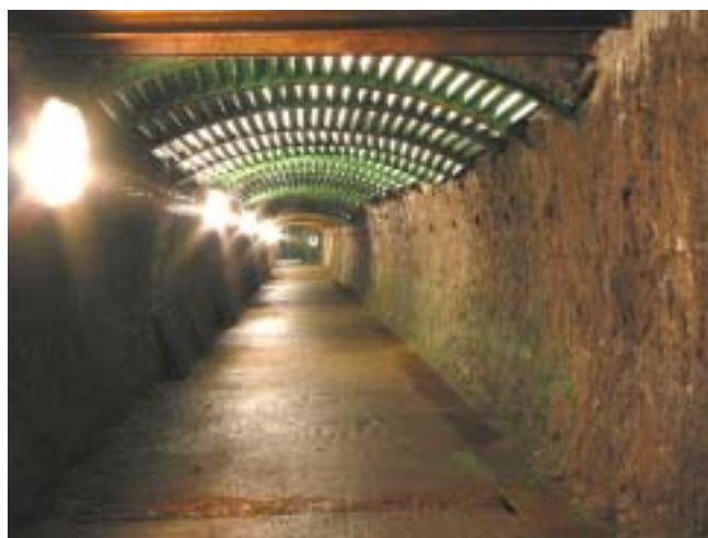
FIG. C-1. View of a part of the storage area in the former mine Bratrství, Jáchymov, Czech Republic.
