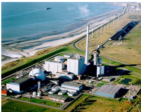
FIG. 1. The Borssele nuclear and coal-fired power plants.
