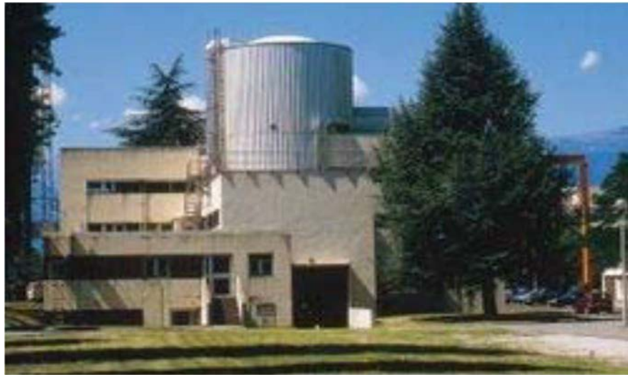
FIG. 69. Exterior view of Siloëtte (photo courtesy CEA).
