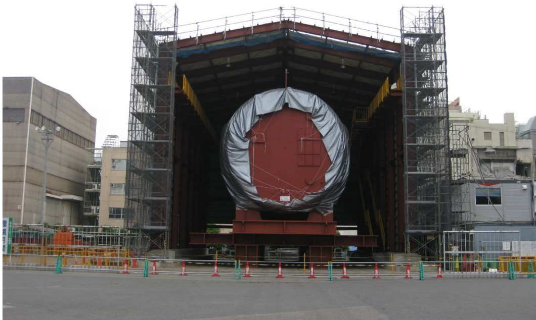
FIG. I-6. Protection of the Reactor pressure vessel (RPV).
