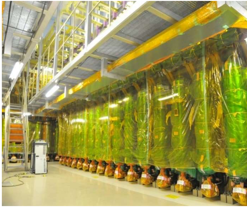
FIG. I-5. Hydraulic control unit of a control rod driving mechanism.
