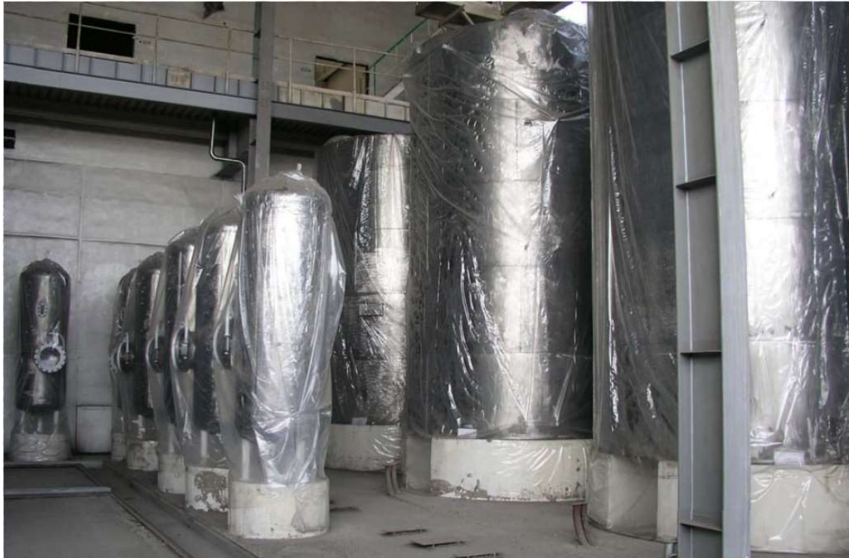
FIG. I-10. Preservation of large component by plastic foil – Tanks and filters in auxiliary building.
