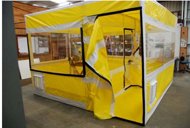
FIG. 4. Example of mock-up training for glove bags and containments (courtesy of Humboldt Bay, USA).
