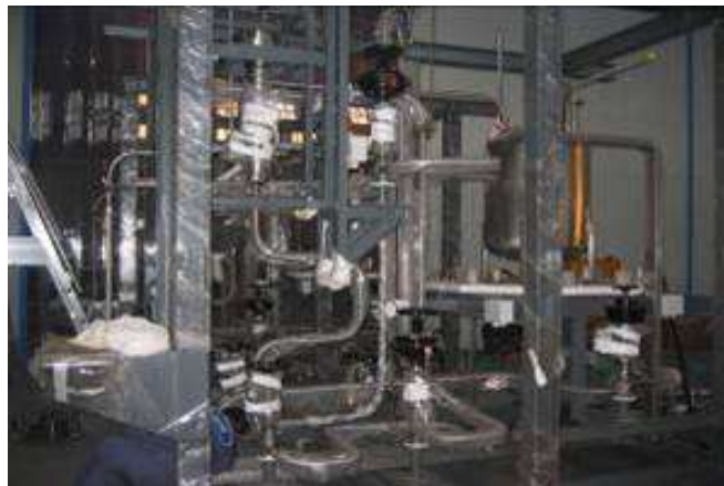
FIG. 2. Sodium Treatment Facility at Creys Malville (courtesy of EDF, France).
