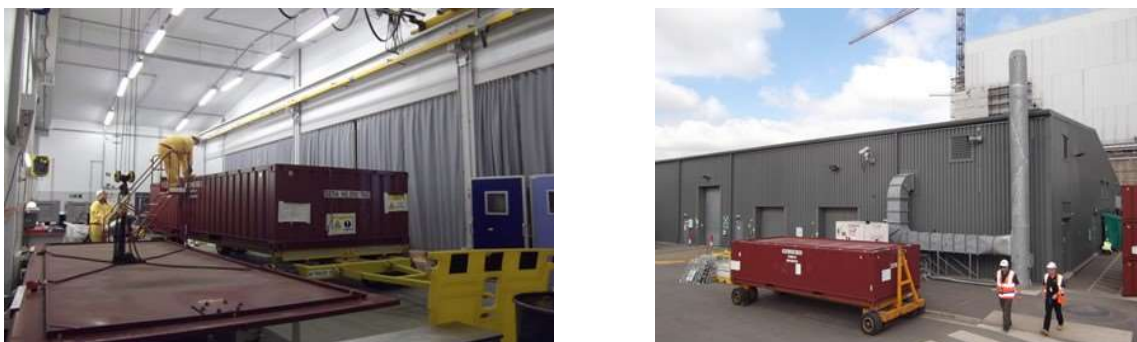
FIG. 8. Waste container constructed for receiving wastes generated during decommissioning (courtesy of Bradwell, United Kingdom).
