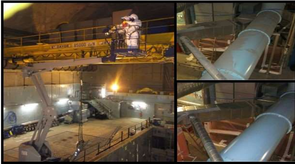
FIG. 12. Chooz A decontamination (2014). Left side – decommissioning of the fuel building. Right side – pipework before and after cleaning (courtesy of Chooz A, France).
