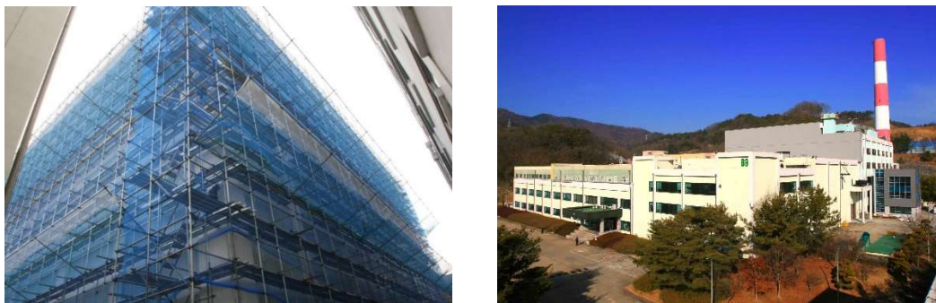
FIG. 3. The construction work for reinforcement of HANARO wall, and the HANARO view after the reinforcement of wall.
