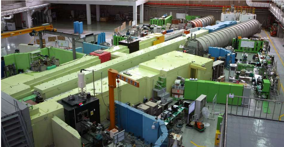
FIG. 2. HANARO cold neutron research facility.
