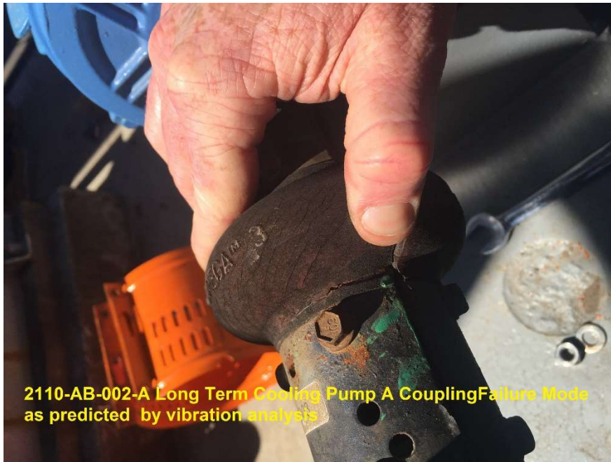
FIG 4. OPAL cooling pump A coupling failure as discovered by vibration analysis.
