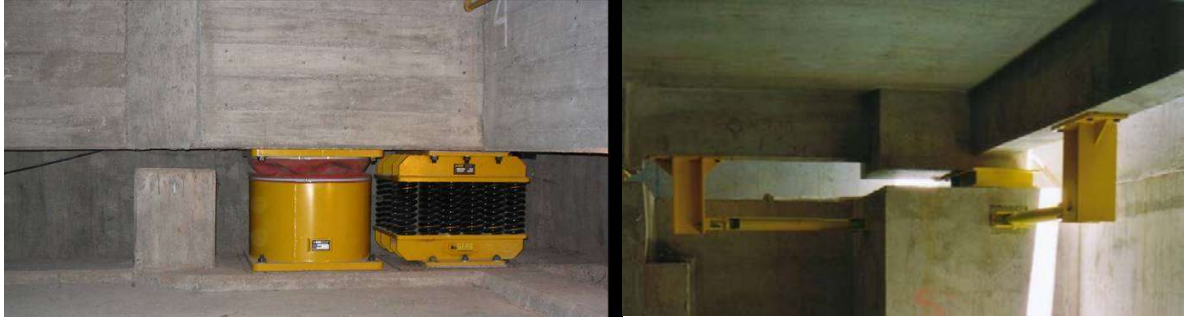
FIG. A.11 Isolators and dampers mounted in parallel
