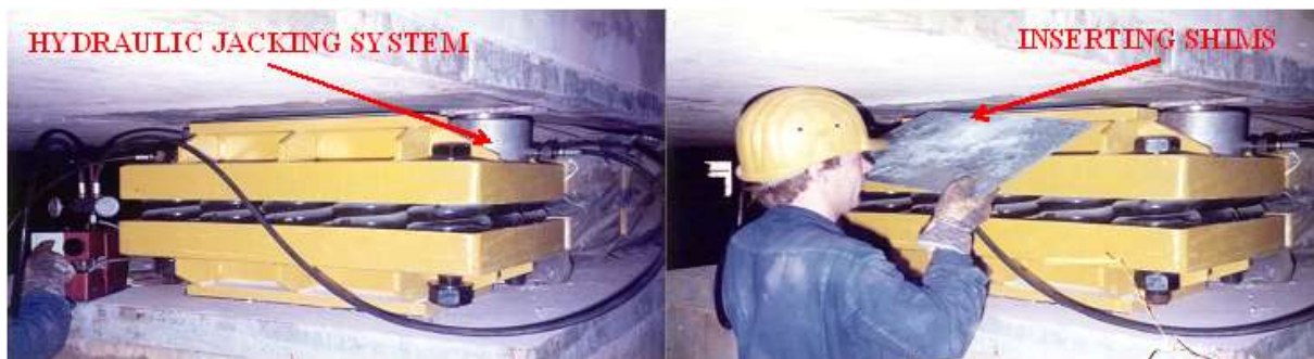
Figure 5. ACCESS, INSPECTION, POTENTIAL ADJUSTMENT AND EXCHANGE OF DEVICES.
