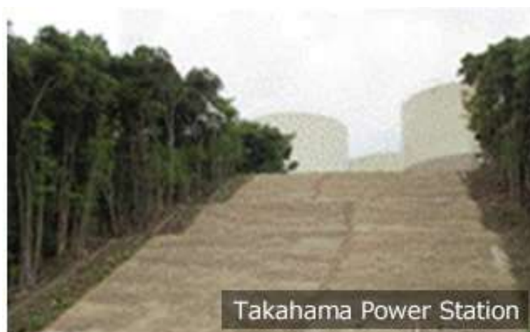
FIG. I-13-8. Image of firebreak zone (Courtesy of © The Kansai Electric Power Company, Incorporated).
