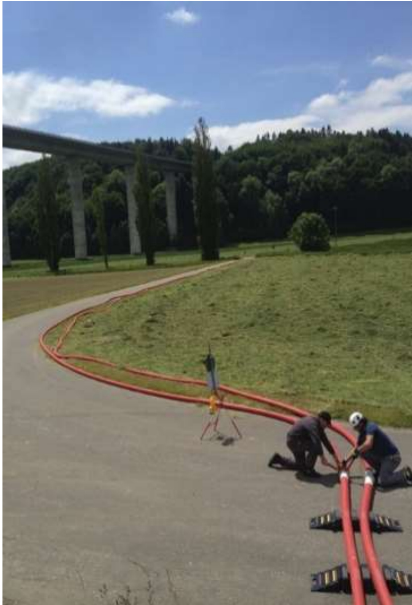
FIG. I-21-8. 2.4 km fire water pipeline.
