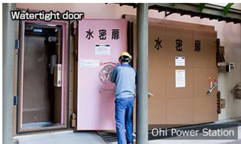
FIG. I-13-7. Example of Watertight doors (Courtesy of © The Kansai Electric Power Company, Incorporated).
