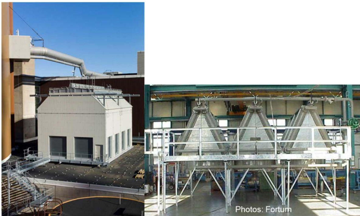
FIG. I-9-7. Independent air-cooled cooling units for decay heat removal from the reactor core and from the spent fuel pools at the Loviisa NPP [Fortum]
