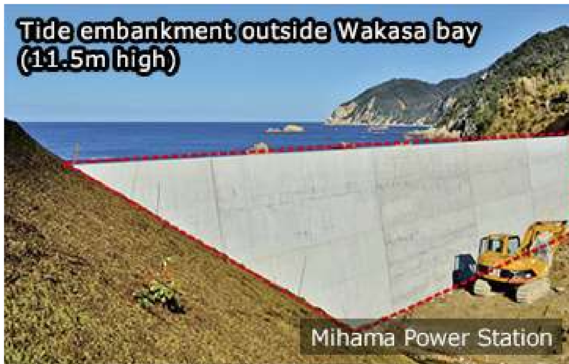
FIG. I-13-6-. Tide embankment at Mihama Power Station (Courtesy of © The Kansai Electric Power Company, Incorporated).
