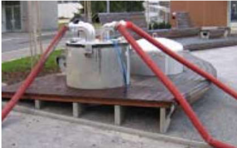
FIG. I-21-5. Cooling water injection point.
