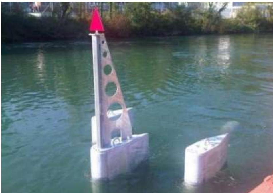
FIG. I-21-4. Protection of the suction pipe (bumper).
