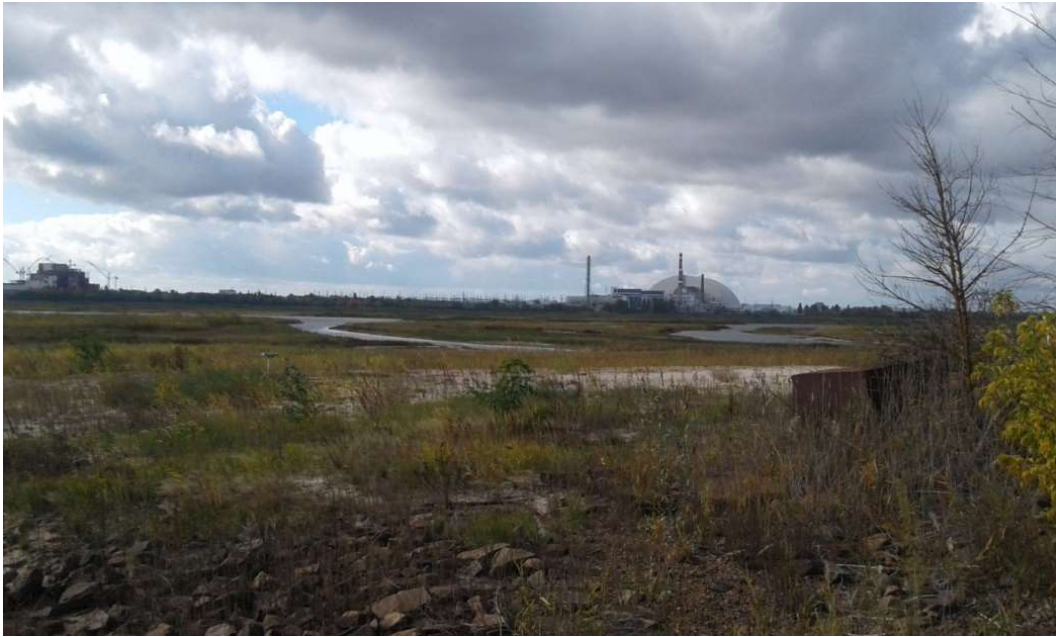
FIG. 58. View on the drained bottom of the cooling pond from the former pumping station (from the northeast corner of the pond, October 2017) (reproduced courtesy of D.Bugai, IGS).
