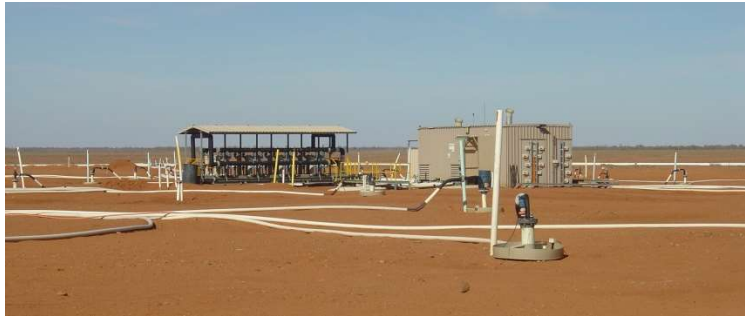
FIG. 4. Uranium in situ leach operation (Beverley, South Australia, courtesy P. Woods, IAEA).
