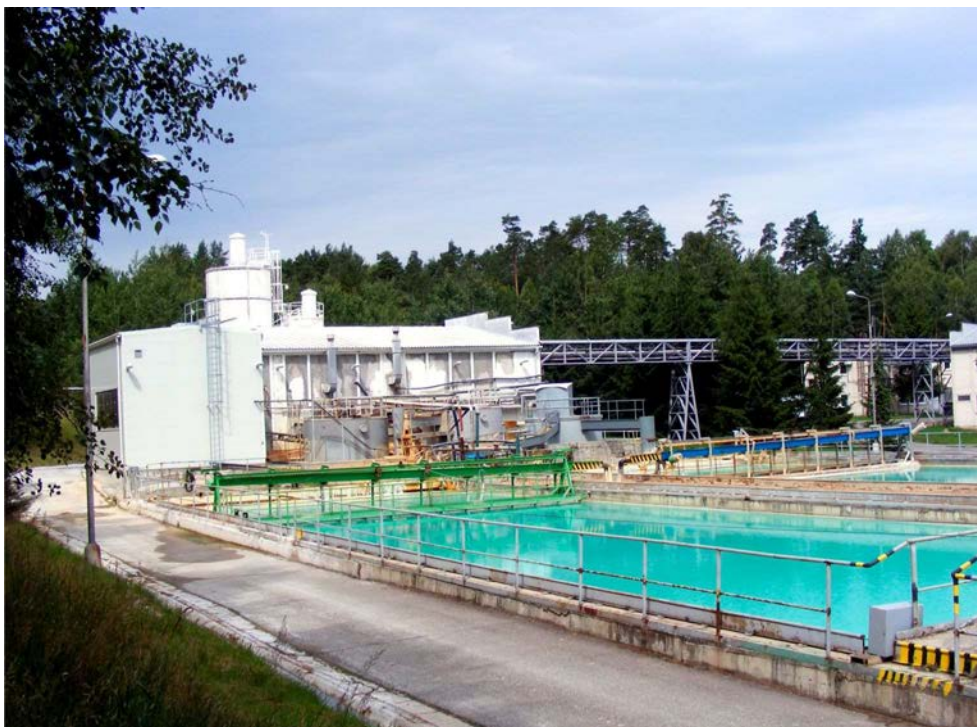
FIG. 10. Neutralization and decontamination station NDS 6 (courtesy of DIAMO s. e.).
