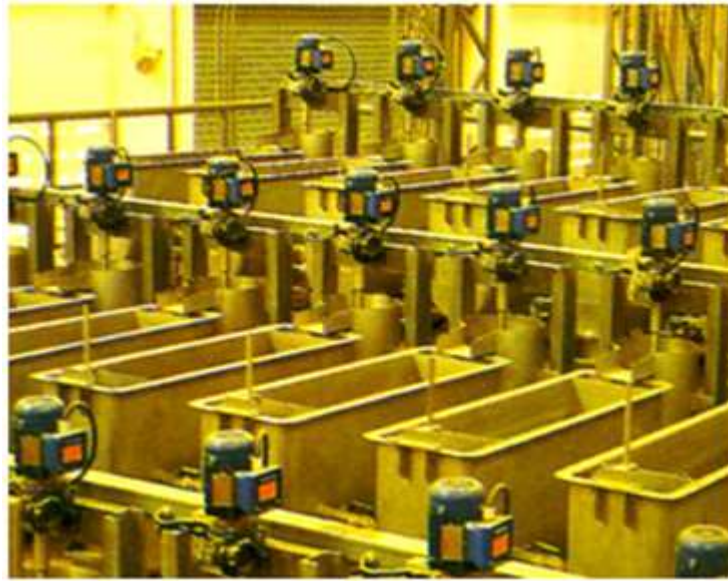
FIG. 6. Pump mix mixer-settlers.
