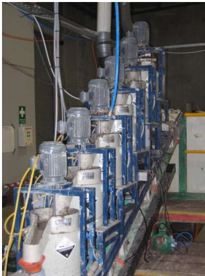
FIG. 8. Atmospheric leach circuit of a pilot plant (courtesy of SGS Pty Ltd).
