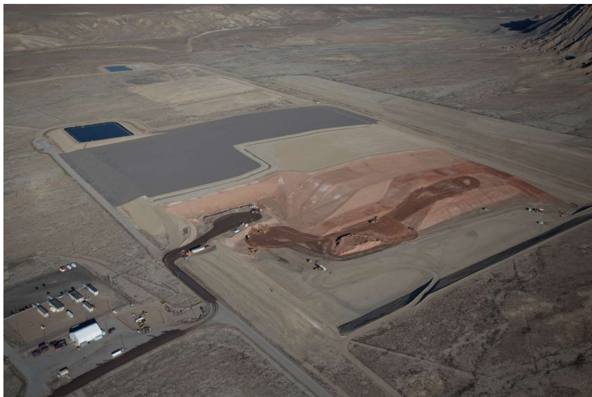
FIG. 4. Crescent Junction disposal site, 2014. From left, final cover (dark grey), interim cover placed (light tan), RRM being placed (red), and excavated cell unfilled.
