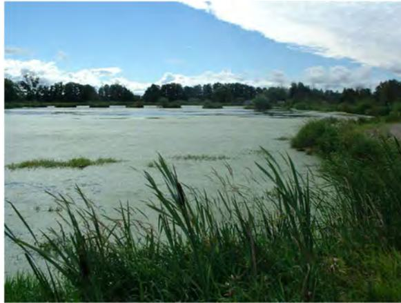
FIG. 21. Ekeby treatment wetland, Eskilstuna, Sweden. The wetland is excavated in natural clay deposits and used as a final 'polishing' step in the wastewater treatment plant in the municipality of Eskilstuna.
