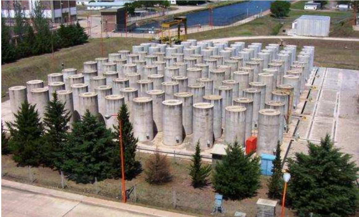
FIG.1. Spent fuel storage silos battery at embalse NPP.
