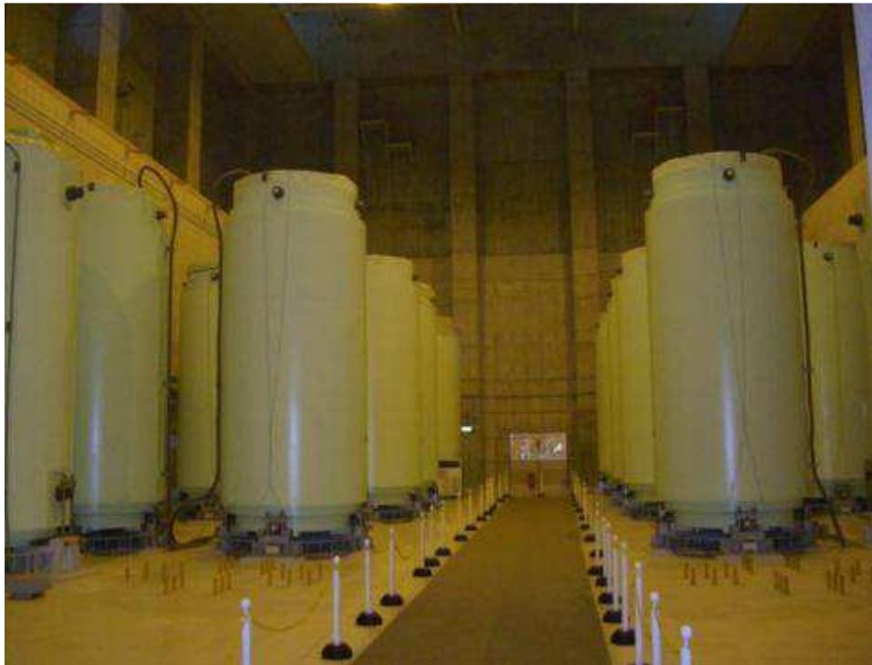
FIG. 1. The air view of storage facility and current state of facility.
