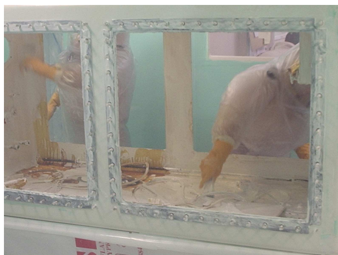
FIG. 8. Progressing the application of fresh tie down coating, to supplement coating already in place, prior to size reduction commencing.
