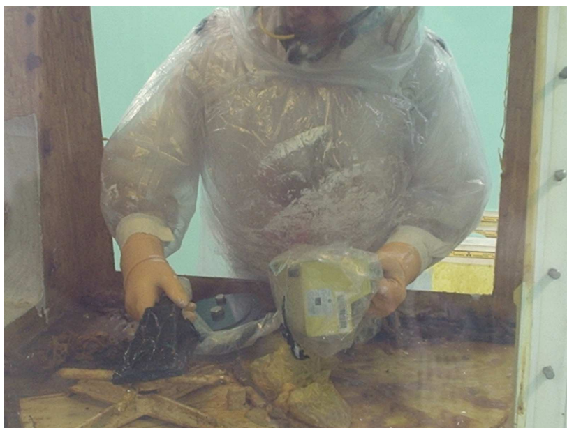
FIG. 14. Monitoring of glovebox interior to check for 'high' areas to target for early removal. NDA analysis had already been used to indicate inventory of the glovebox. Swab samples taken at this point would be sent for analysis to confirm activity 'fingerprint'.
