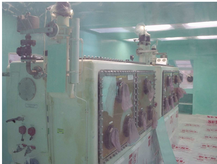
FIG.12. Interior of containment prior to commencing size reduction. Temporary fluorescent lighting (with internal battery backup in case of power loss) installed over roof lights. Floor covered by several layers of non-slip sheeting. Strippable coating (tinted) applied. All 'low active' glovebox peripherals removed.
