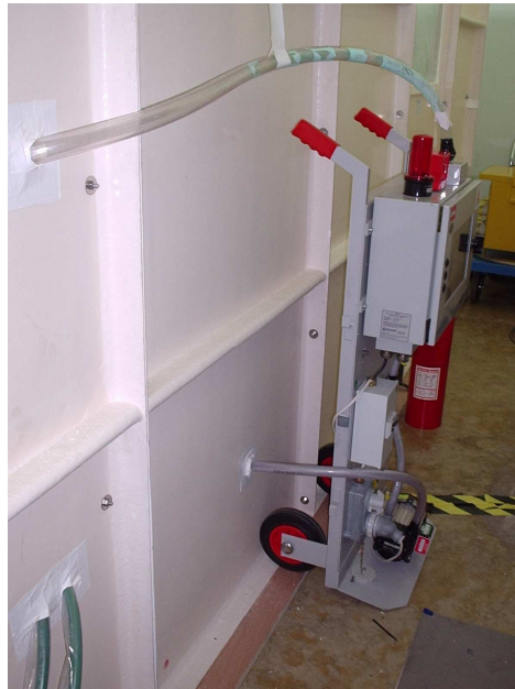
FIG. 11. Temporary air particulate monitors installed to check for activity in the containment change areas.
