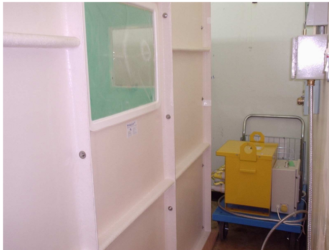
FIG.9. Temporary low voltage transformer to provide tooling supplies.
