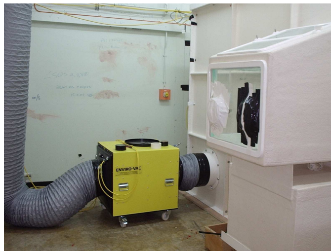
FIG. 10. Temporary air handling unit to provide extract from containment (via pre-filter and HEPA filters) and maintain set airflow rate across all barriers.
