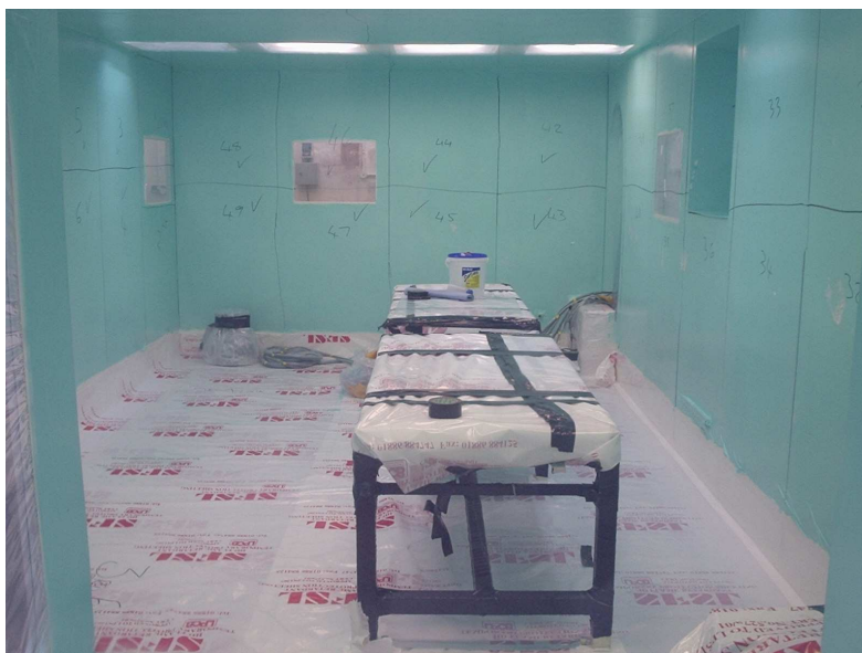
FIG. 15. Gloveboxes removed, stands decontaminated and covered for disposal as low level waste, containment floor sheeting layers removed to expose an uncontaminated layer, and Modular containment interior marked out and confirmed free of contamination. After this point the tie-down coating and joint tape will be removed, and the containment dismantled for re-use elsewhere.
