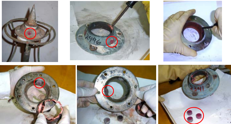
FIG. 5. Radioactive lightning rod Helita: dismantling operations.
