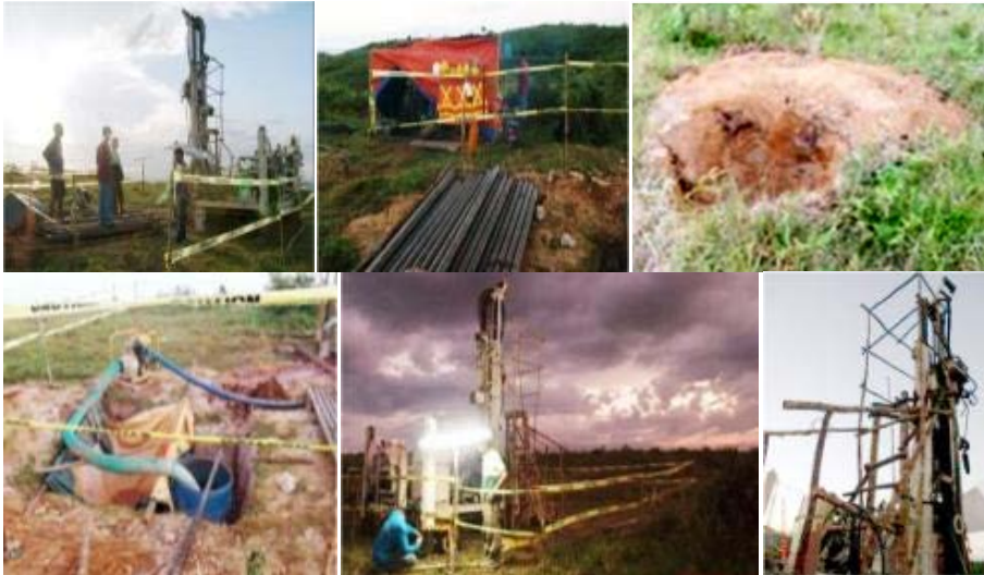
FIG. 12. Drilling of a 100 m deep investigation borehole.
