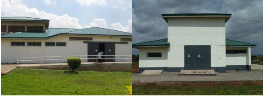
FIG. 1. Centralized waste processing and storage facility.
