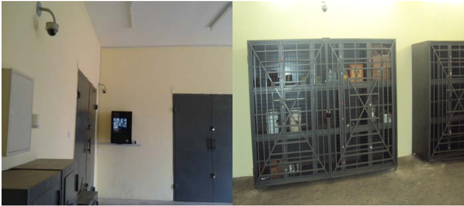
FIG. 2. Physical protection systems in the storage facility and storage cages for the radioactive waste materials.
