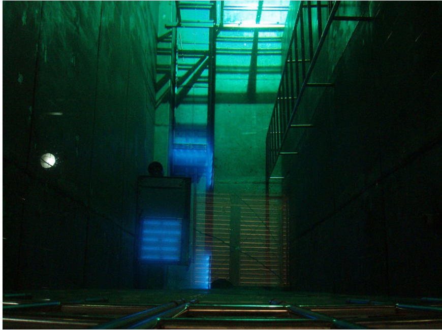
FIG. 7. Wet storage of Category 1 sources in the water pool.
