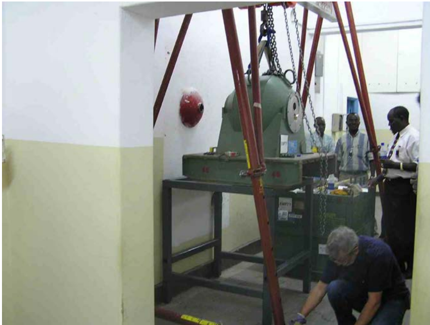
FIG. 55. Rigging and lifting of a teletherapy head.
