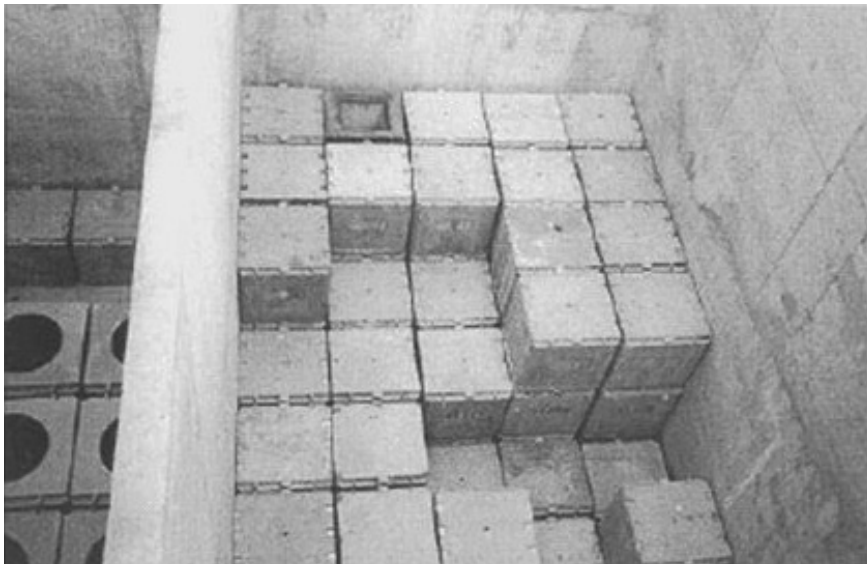
FIG. 77. The concrete vaults used to house concrete boxes.
