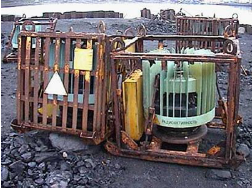
FIG. 74. Inadequate area storage of RTGs.
