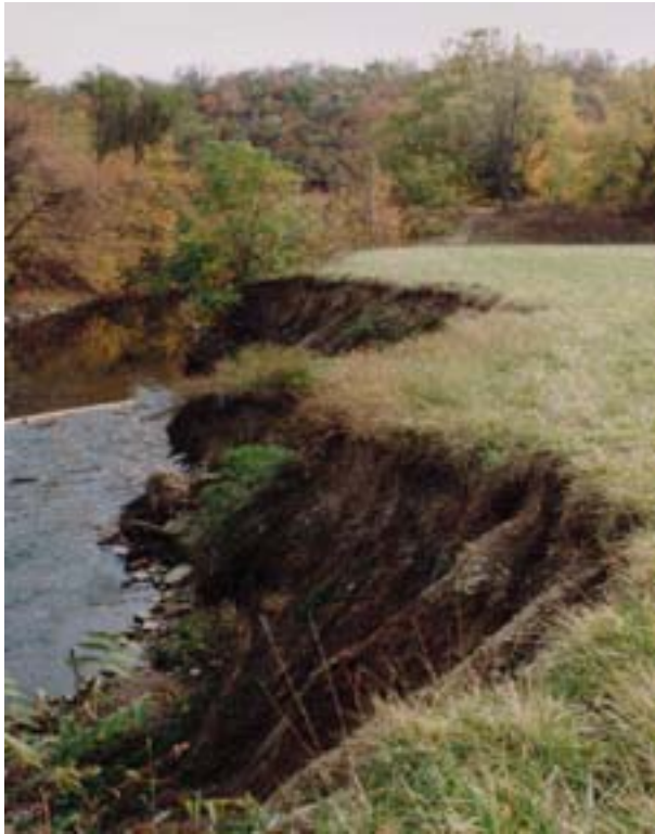
FIG. 10. Stream meandering leading to bank failure.
