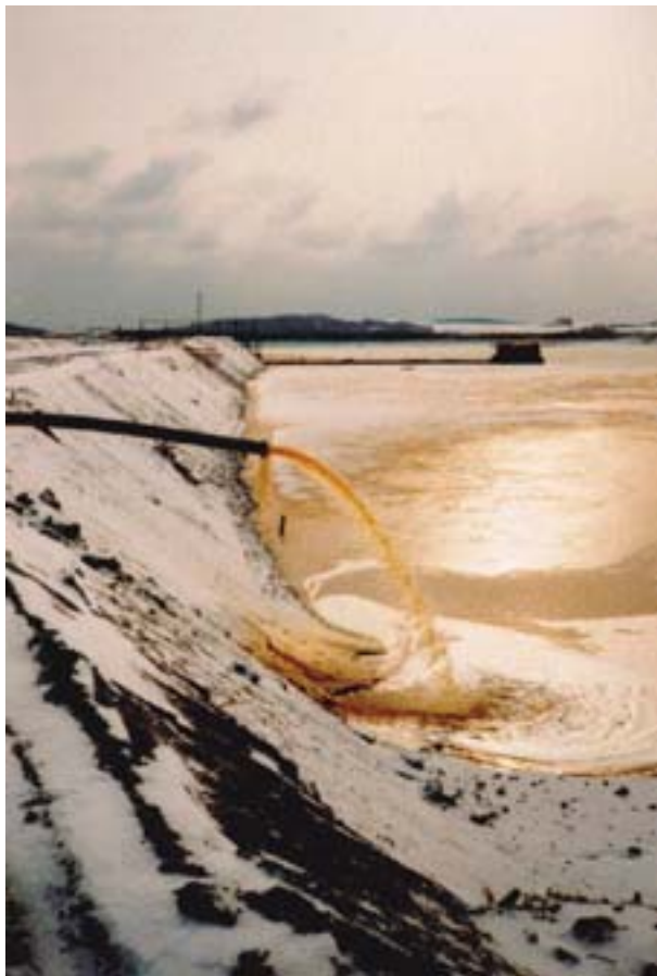
FIG. 2. Tailings pond in operation.
