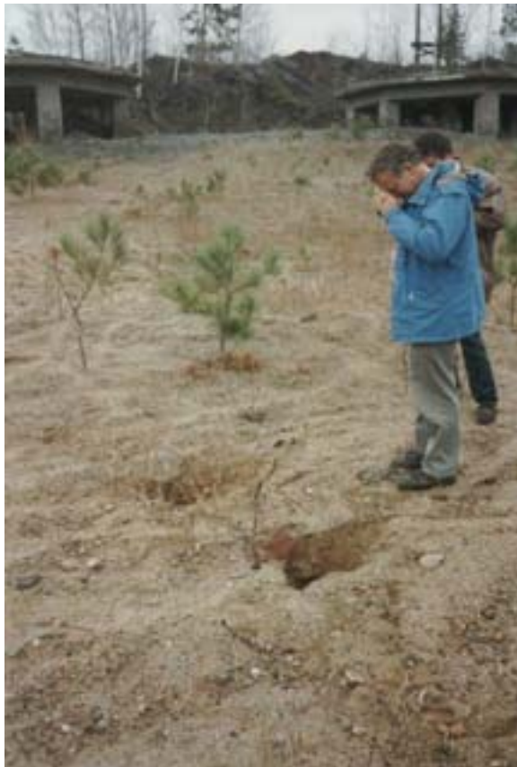
FIG. 9. Hole in a tailings cover caused by decomposing wood.
