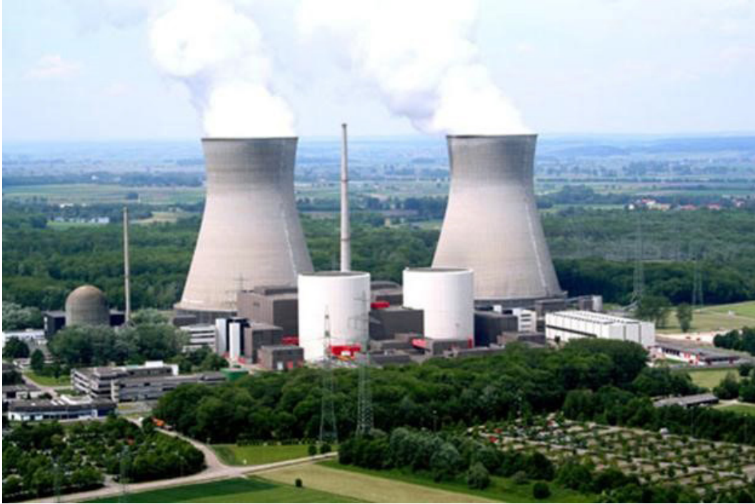
FIG. 18. The Gundremmingen NPP site. The smaller Unit A currently under decommissioning is on the left, next to the two operating units B and C (centre) (photo courtesy of RWE Power AG and PreussenElektra).
