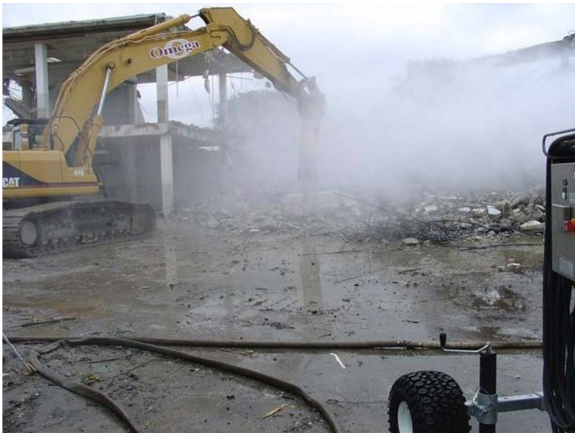
FIG. 12. Fine mist sprays during demolition (photo courtesy of Omega III LLC).
