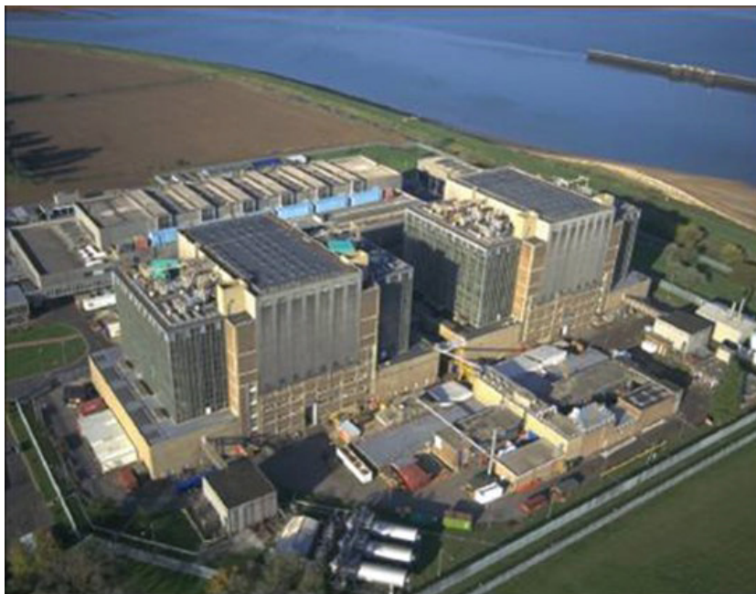
FIG. 8. The two Magnox reactors at the Bradwell site, UK (photo courtesy of NDA).
