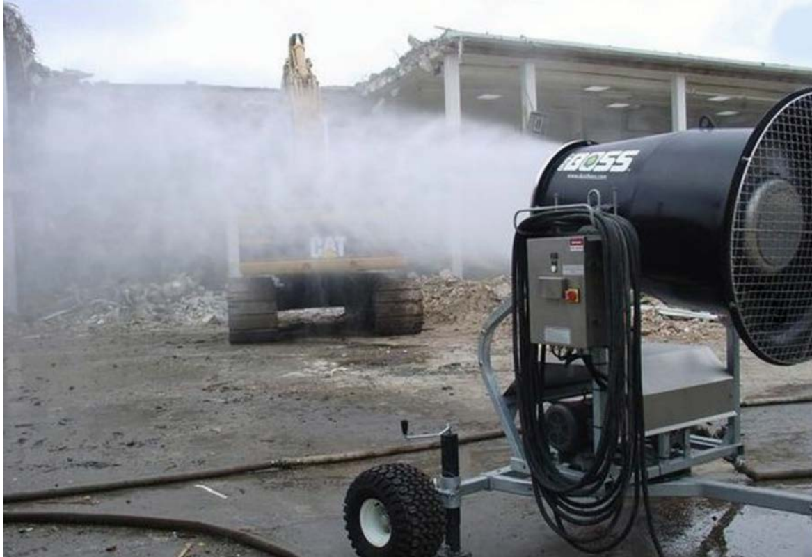
FIG. 13. Water cannon used for fine mist spraying (photo courtesy of Omega III LLC).
