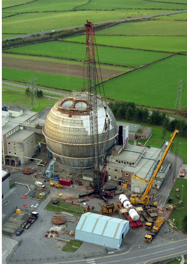
FIG. 14. Removal of steam generators from the top of the Windscale AGR, UK (photo courtesy of NDA).
