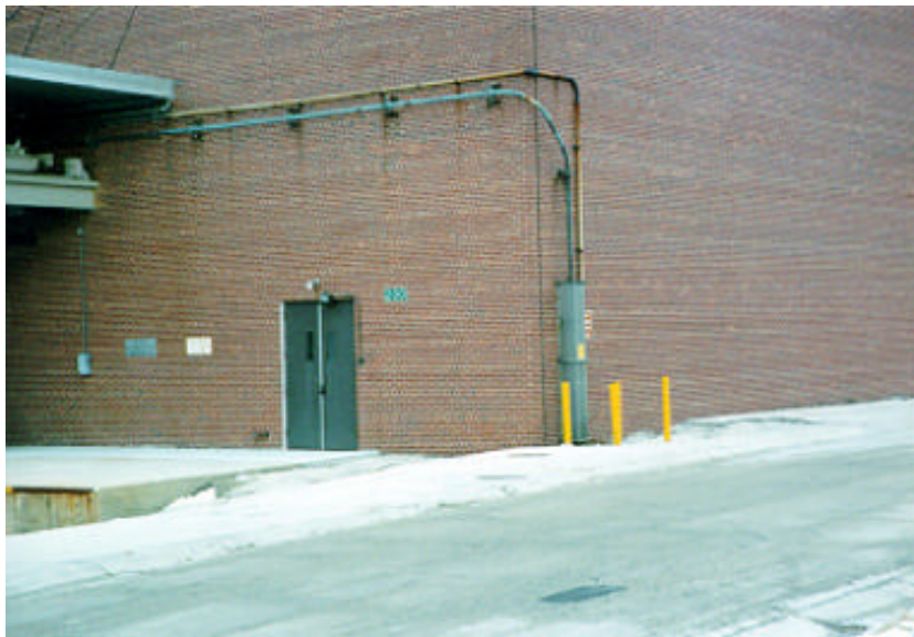
FIG. 15. Building 200/205 pneumatic transfer tube (photo courtesy of ANL).
