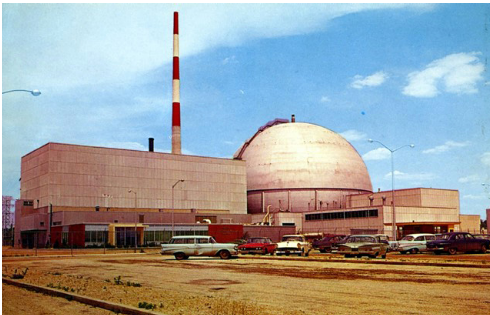
FIG. 17. The Dresden-1 nuclear reactor, Illinois, USA (photo courtesy of Exelon Corporation).
