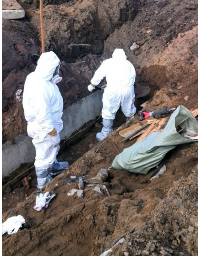
FIG. 16. Opening and removal of contaminated ventilation system in Building 53, Moscow, Russian Federation (photo courtesy of VNIINM)
