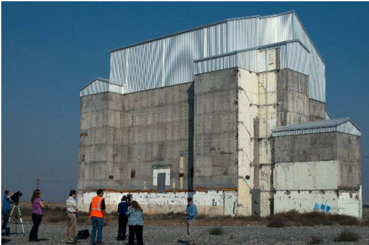
FIG. 7. Safe enclosure completed at the Hanford F reactor, which operated from 1945 to 1965 and was placed in interim safe storage in 2003 (photo courtesy of the United States Department of Energy (DOE)).
