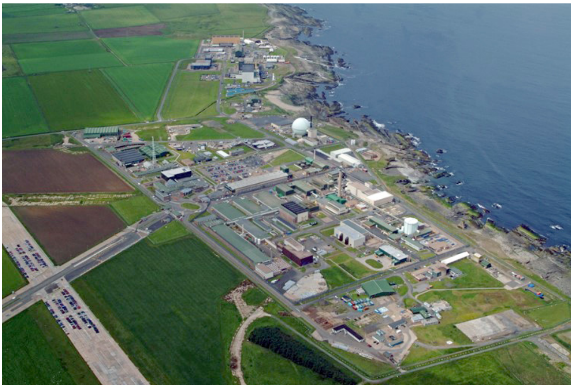
FIG. 3. The Dounreay site, UK (photo courtesy of the UK Nuclear Decommissioning Authority (NDA)).
