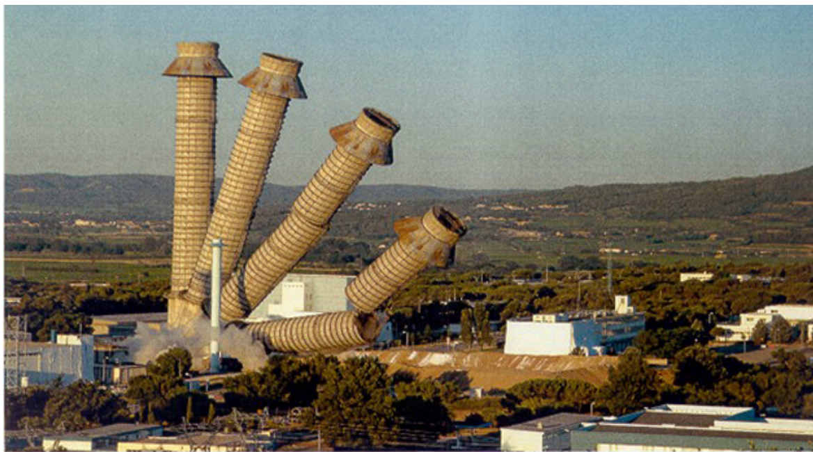
FIG. 9. Stack dismantling at the G1 reactor, Marcoule, France (photo courtesy of CEA Marcoule).
