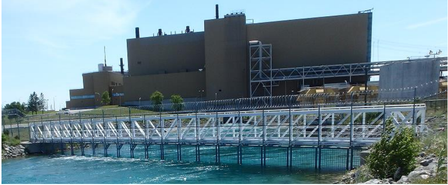
FIG. 38. Marine barrier anchored to the shoreline. (Courtesy of the Canadian Nuclear Safety Commission.)
