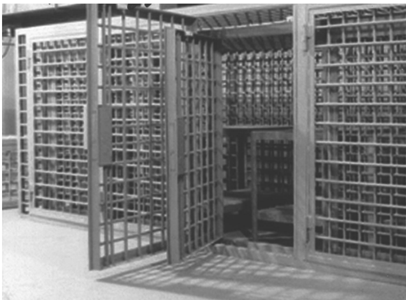
FIG. 35. Double layer steel cage for nuclear material storage. (Courtesy of Sandia National Laboratories.)
