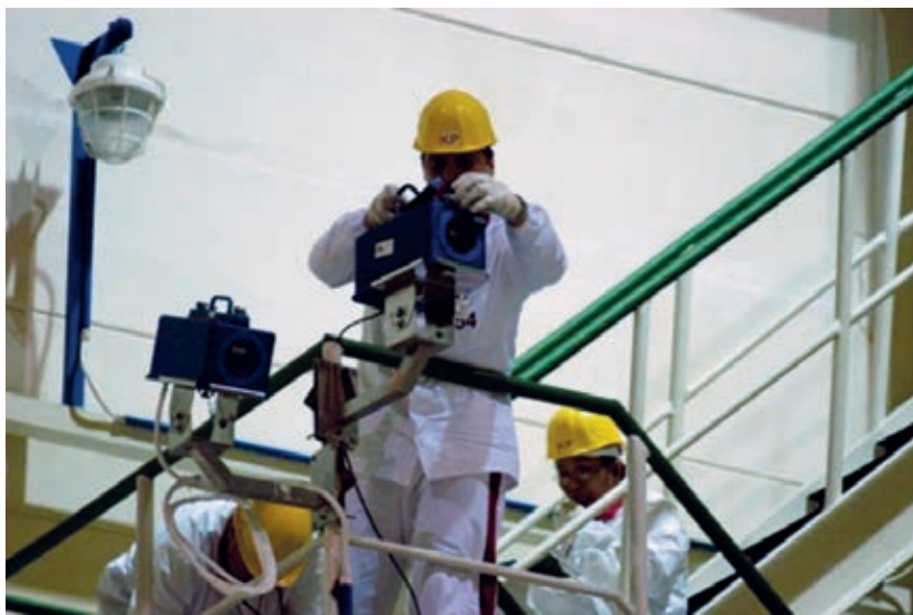
FIG. 10. Installation of a surveillance system.
