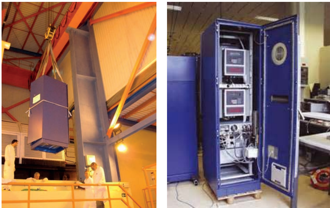
FIG. 8. A facility operator supporting the installation of IAEA equipment racks.
