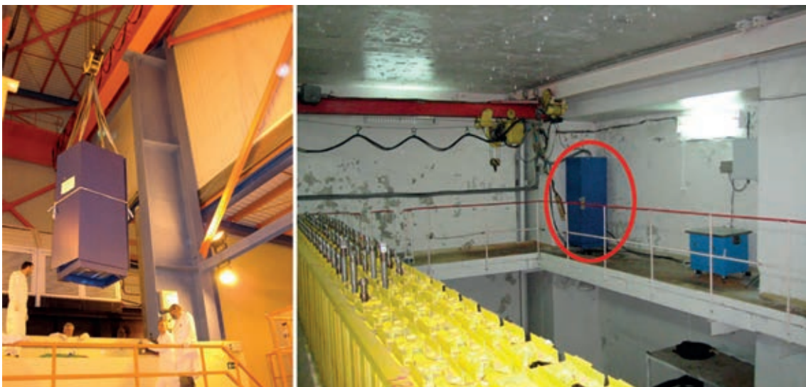
FIG. 11. Receipt and installation of IAEA equipment racks.
