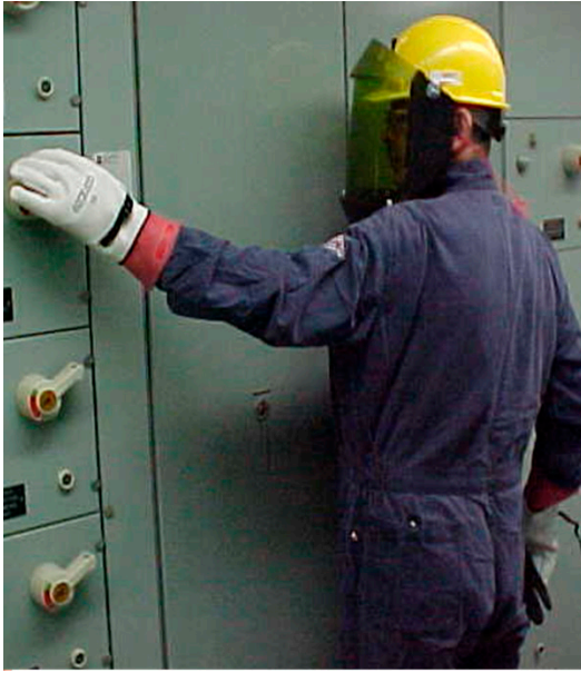
FIG. 57. Arc flash related improvements at Ontario Power Generation, including changes in manual switching practices, new remote racking tools and exclusion boundary shields (courtesy of Ontario Power Generation).
