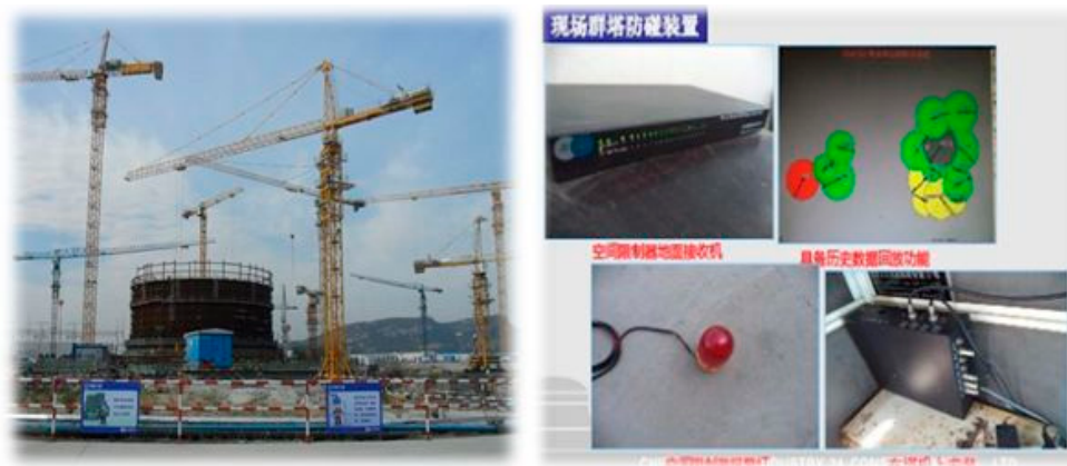
FIG. 28. Crane collision warning system components (courtesy of the China National Nuclear Corporation).
