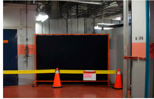
FIG. 57. Arc flash related improvements at Ontario Power Generation, including changes in manual switching practices, new remote racking tools and exclusion boundary shields (courtesy of Ontario Power Generation).
