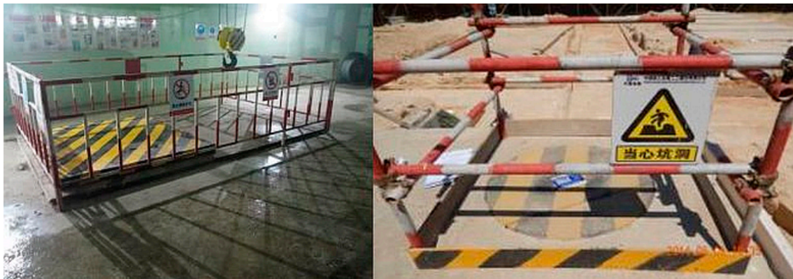
FIG. 52. Hole protection standards from the occupational safety and health manual (courtesy of the China National Nuclear Corporation).
