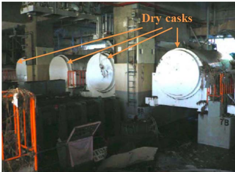
FIG. 3 Dry Casks; photographed March 17, 2011 (copyright: TEPCO, [3]).
