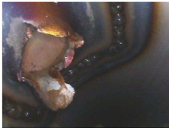
FIG. 3. Damaged make up feed water pipe.
