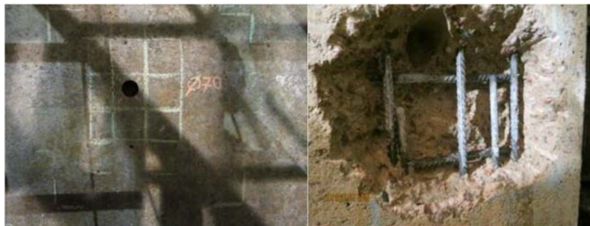
FIG. 6. Concrete structure testing.
