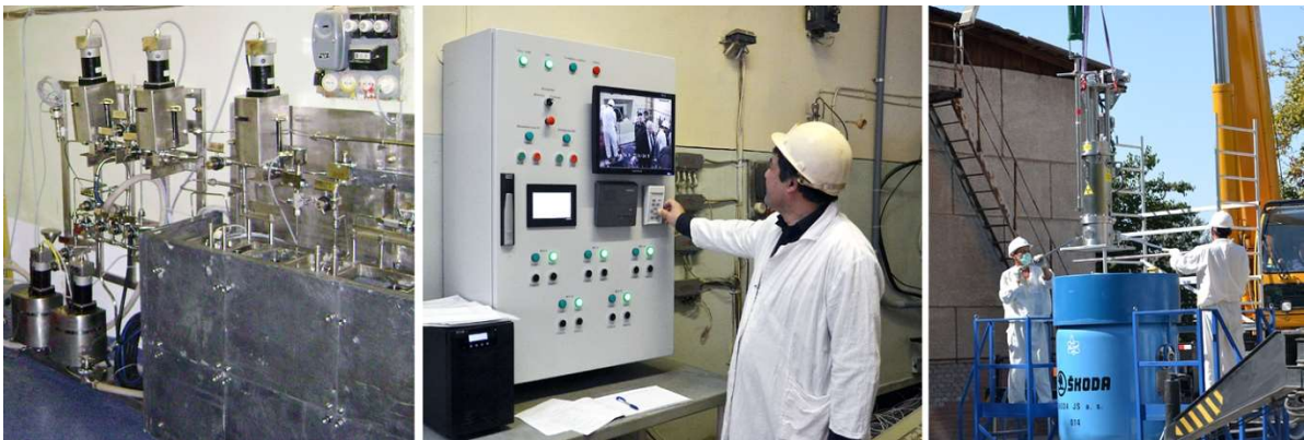
FIG. 3. Equipment for preparation of INN-3M LSNF removal.
