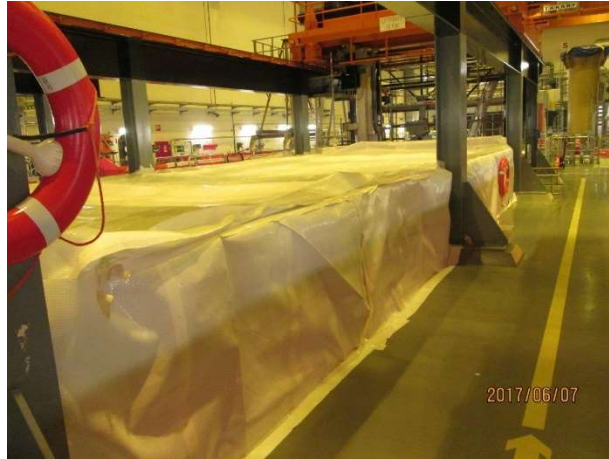
FIG. 2. FME-covering of the unloading pool.
