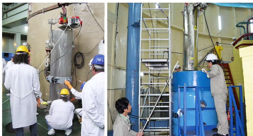
FIG. 2. Loading canisters with liquid SNF into SKODA VPVR/M through the transfer cask.
