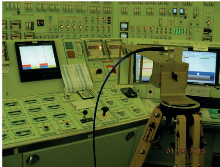
FIG. II-2. Emissions site survey.
