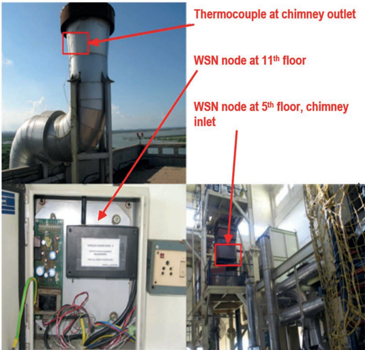
FIG. 7. Wireless sensor network (WSN) deployed at the Safety Grade Decay Heat Removal Loop in Sodium facility.
