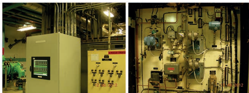
FIG. II-1. Various aspects of plant equipment installation identified during walkdown.
