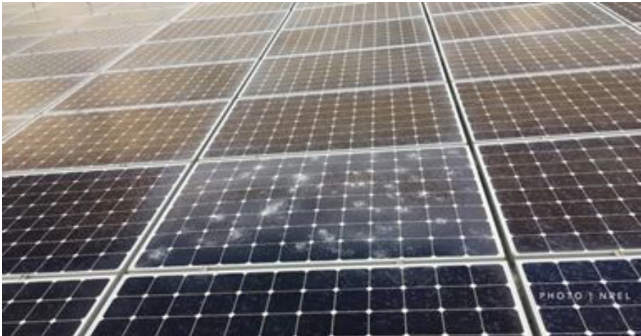
FIG. 14. Just one photovoltaic panel out of more than 3000 was damaged at Golden, Colorado, United States of America, after the hailstorm on 8 May 2017. (Reproduced with permission courtesy of the National Renewable Energy Laboratory.)
