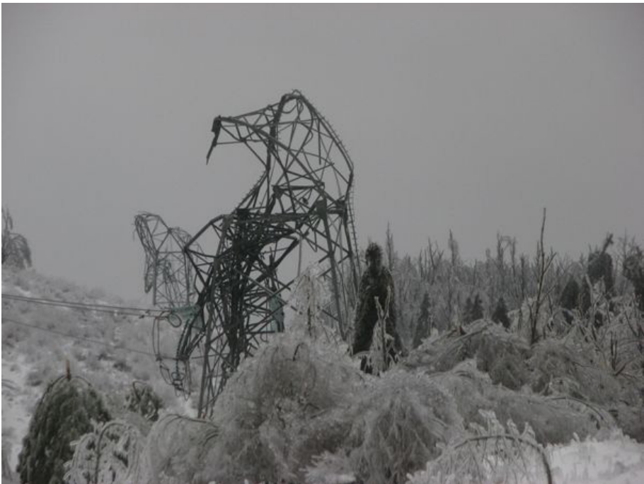
FIG. 15. Damage caused by glaze ice on the 400 kV Beričevo-Divača power line, Slovenia, February 2014. (Courtesy of the Slovenian transmission network operator, ELES.)
