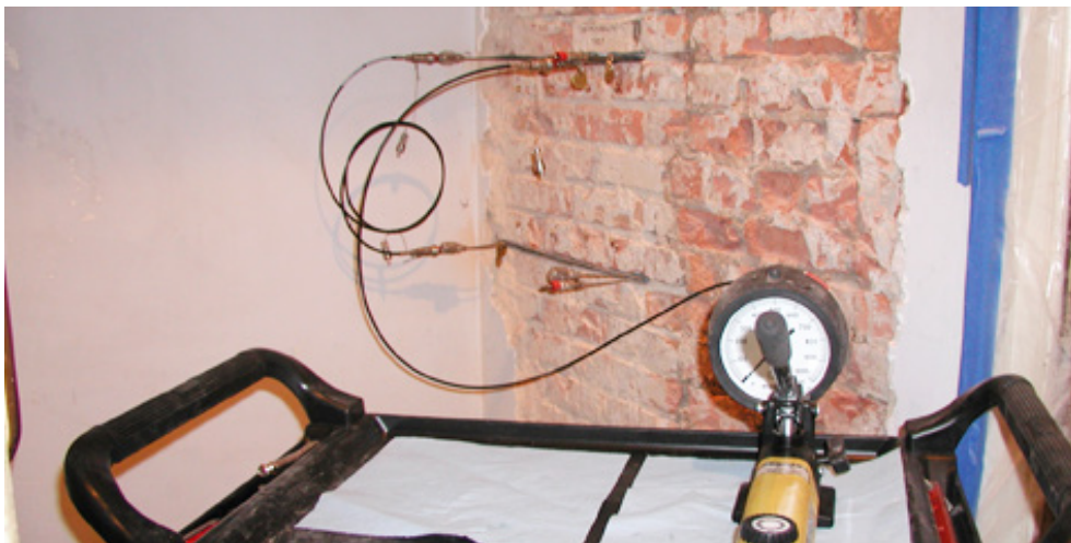
FIG. 116. In situ deformability test using two flatjacks (courtesy of Feld, Kaminetzky & Cohen, P.C.).
