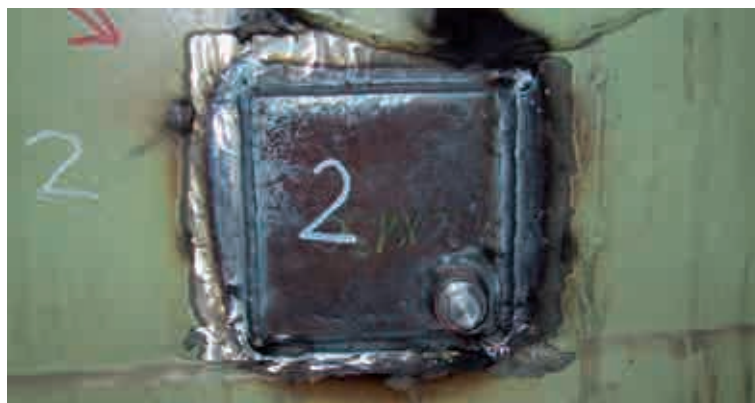
FIG. 161. Repaired liner.
