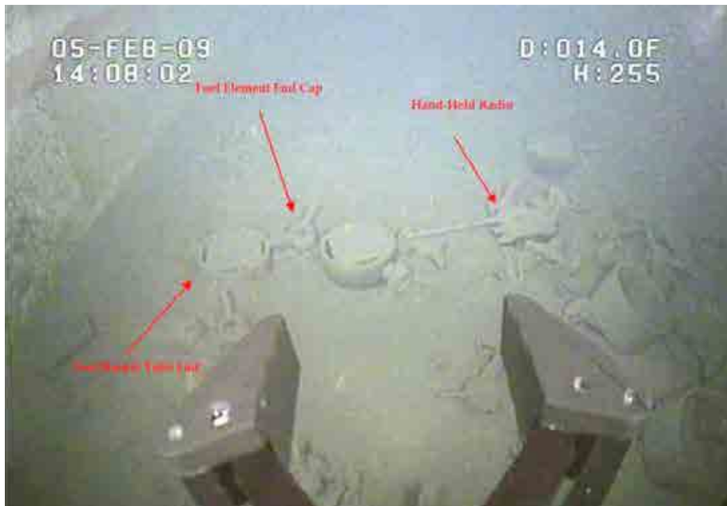
FIG. 60. Remotely operated vehicle photograph of debris in spent fuel pool during decommissioning work (courtesy of Atlantia Marine).
