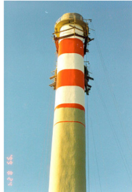
FIG. 204. Condition after repair.
