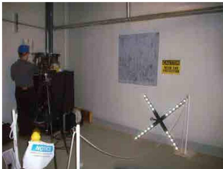
FIG. 130. Digital image correlation cameras and inspection location on outside containment wall [481].
