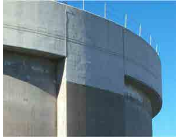
(b) After repair, 2008.
