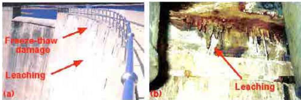
FIG. 32. Examples of leaching: (a) a dam with freeze-thaw damage and leaching; (b) NPP tendon gallery leaching [9].
