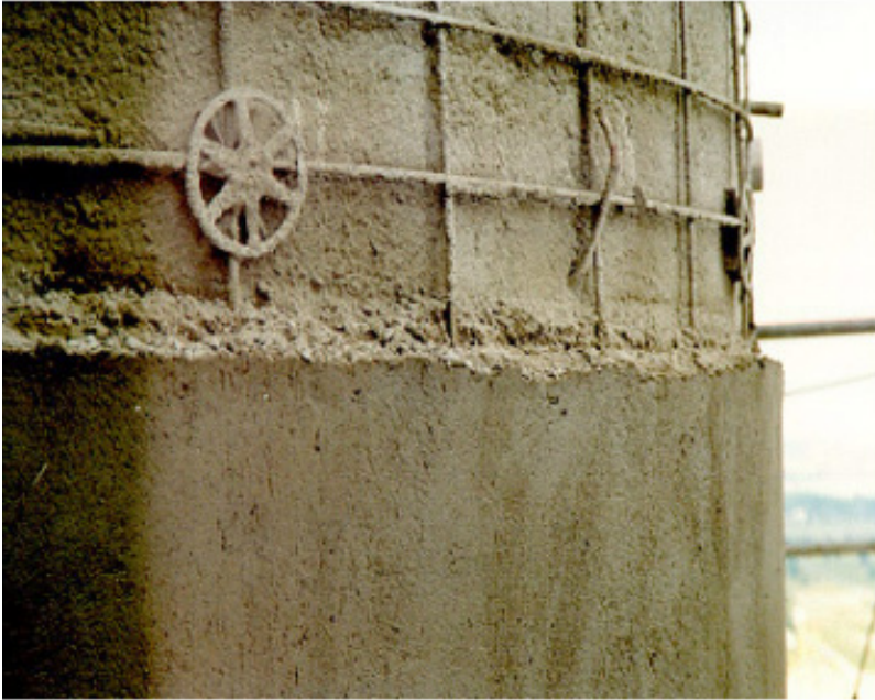
FIG. 203. Condition during repair.
