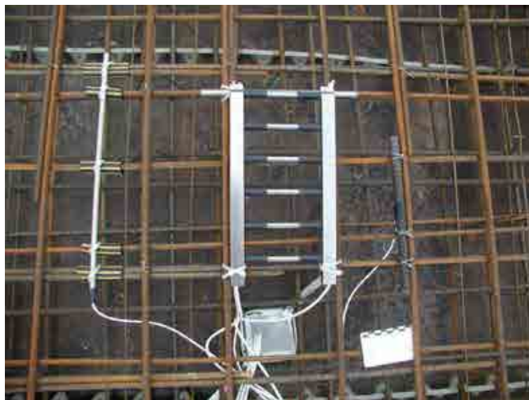
FIG. 140. Anode ladder system installation for corrosion monitoring [495].
