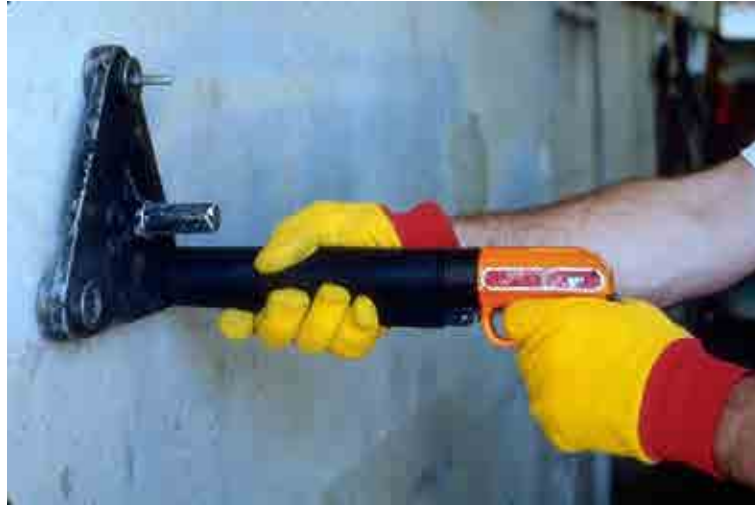
FIG. 89. Windsor probe test technique [395].
