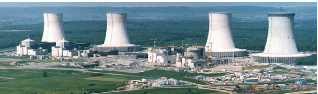
FIG. 9. Natural draft cooling towers at Cattenom NPP, France (courtesy of Hamon Thermal Europe SA).
