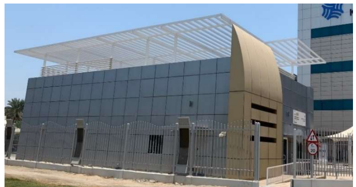
Figure 25. Building hosting the UAE SSDL in Abu Dhabi
