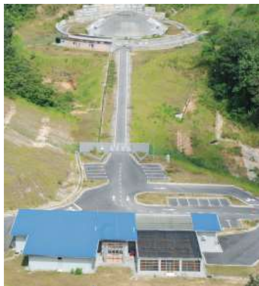
Aerial view of the gamma greenhouse.
