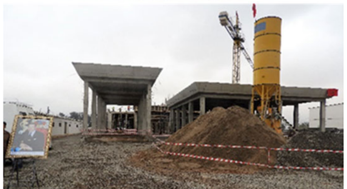
Layout of the Mediterranean fruit fly mass-rearing and fly emergence and release facilities (top) and construction site in April 2018 (bottom).
