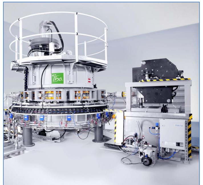
The new rhodotron electron accelerator installed at Aerial in 2019.
