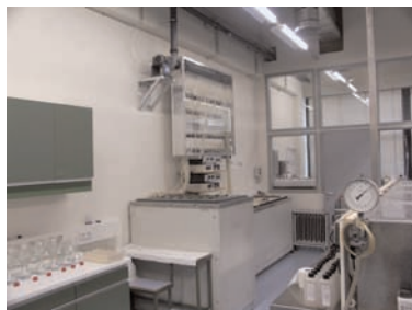
Two tritium electrolysis systems with wall-mounted gas bubblers and safety gas dilution system.
