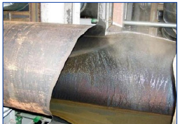
FAC caused pipe rupturing at the Mihama NPP in 2004. (Photo: http://www.corrosion-doctors.org )
