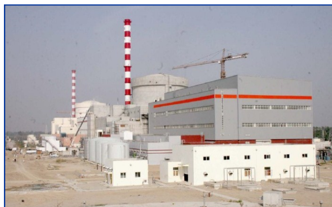
Unit 1 and 2 of the Chasma Nuclear Power Complex, Pakistan. (Photo: PAEC)
