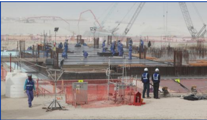
Member States can request a CORR Mission prior to starting major construction. (Photo: ENEC)
