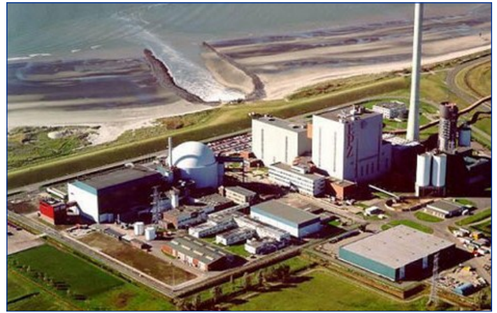
Borssele Nuclear Power Plant in the Netherlands. (Photo: TRACTEBEL Engineering)
