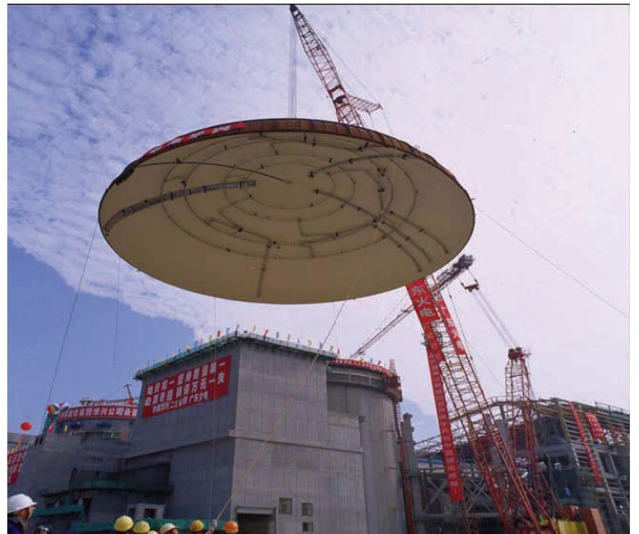
Lifting the dome module into place at Lingao-4 in China
