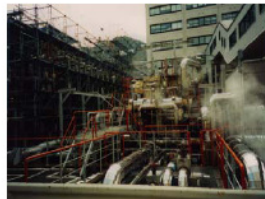
Operating plant: Ohi, Japan
