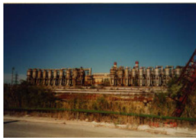
Evaporators at Aktau, Kazakhstan
