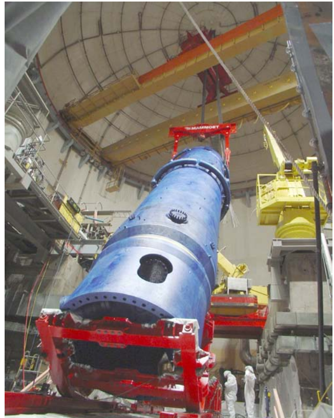
A view of steam generator replacement: steam generator rigging inside a containment
