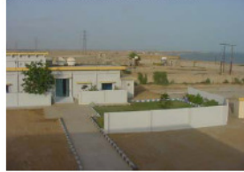
SWRO Plant at KANUPP, Pakistan
