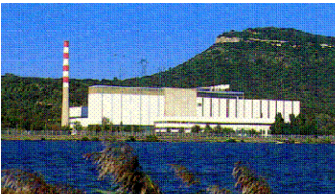
Figure 2. Prototype 250 MW(e) Fast Breeder Reactor Phénix (Credit: CEA/EdF)
