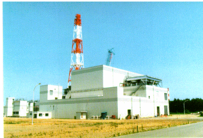
Figure 1. JAERI's High Temperature Engineering Test Reactor has the capability to operate at a core outlet temperature of 950 °C and is utilized to investigate technologies for advanced HTGRs, to demonstrate nuclear process heat applications, and to serve as an irradiation test facility for high temperature research activities (Courtesy of Japan Atomic Energy Agency)
