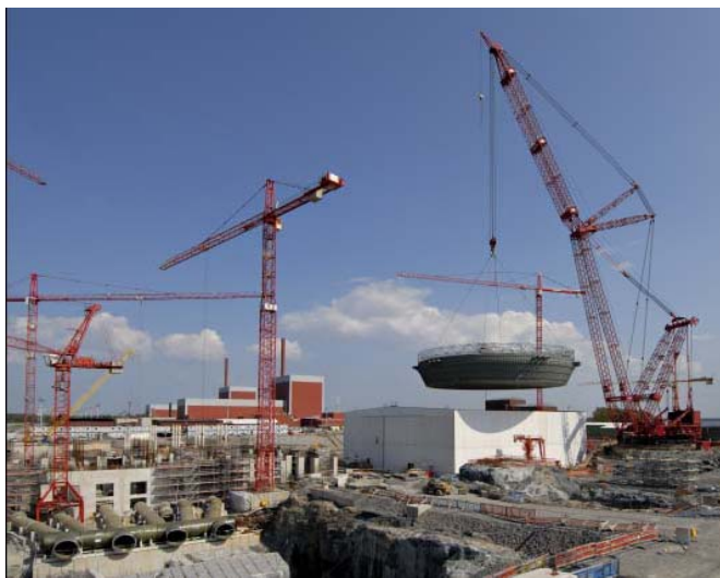
Figure 1. Construction of the European Pressurized Water Reactor in Finland — Positioning of the bottom part of the metallic liner on the base slab (May 2006; credit: Framatome ANP)
