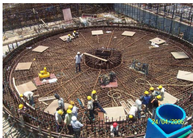
Figure 1. Construction of the Prototype Fast Breeder Reactor (PFBR) at Kalpakkam, India — Reactor Vault Base Preparation (April 2006; Credit: IGCAR)
