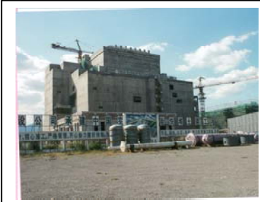
Chinese Experimental Fast Reactor (CEFR) under construction, 2004. (Credit: CIAE)
