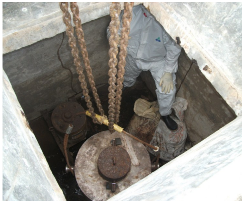
Two irradiators had been stored for years under unsafe and insecure conditions in a bunker. While recovering them, a radium-contaminated capsule was also found in the bunker. All of them were removed, after which the bunker was cleaned and closed.
