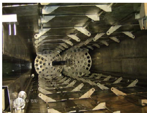
Figure 3 – All spools installed
