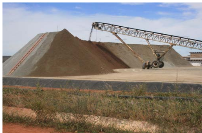
Building a heap leach pile at Caetite mine, Brazil
